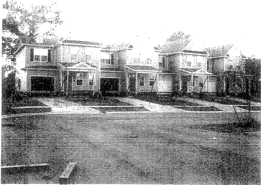
Bandolier Circle, 1357, All Support Beams Installed, 09/12/08
